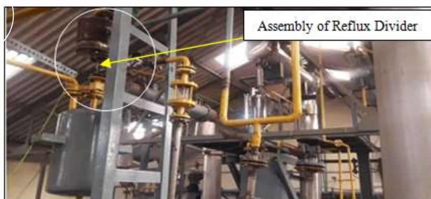
Fig. 2 Actual Reflux divider in the distillation process.
