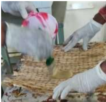
Fig.6 Applying Epoxy on the fiber
